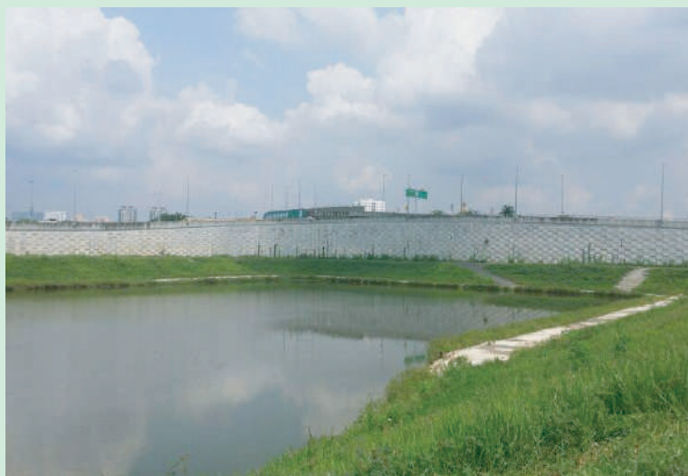
Kolam takungan banjir Puah, Selangor
