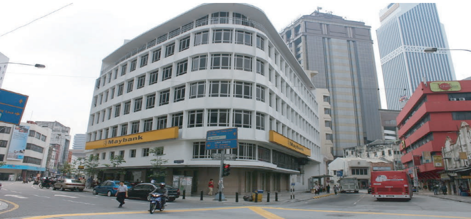
Maybank, Jalan Tun H.S Lee
